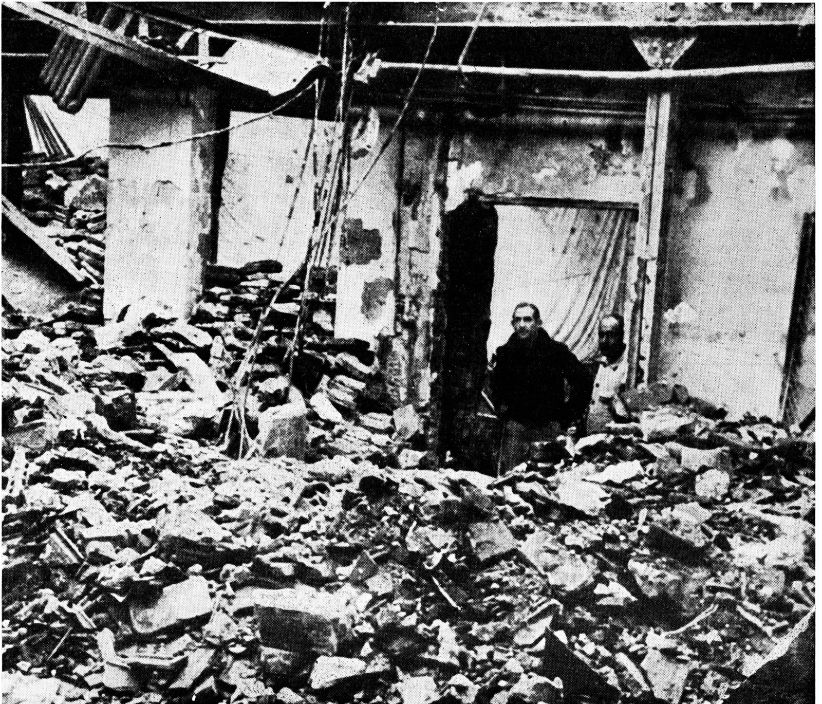
One of Franco's recent projects to restore Spanish culture. Only a pile of rubble remained after fascist aviators bombed this public building in Madrid.
