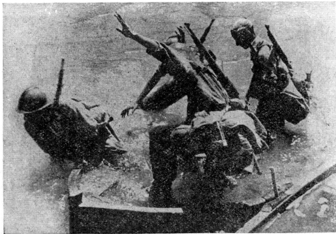
SINKING. One of the pontoons, used to bridge the Ebro during the attack, founders.
