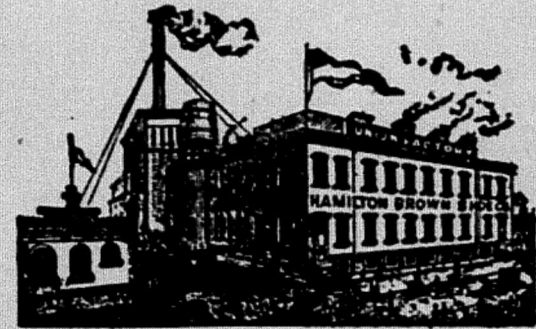
New Union Factory on Randolph, near Jefferson.
