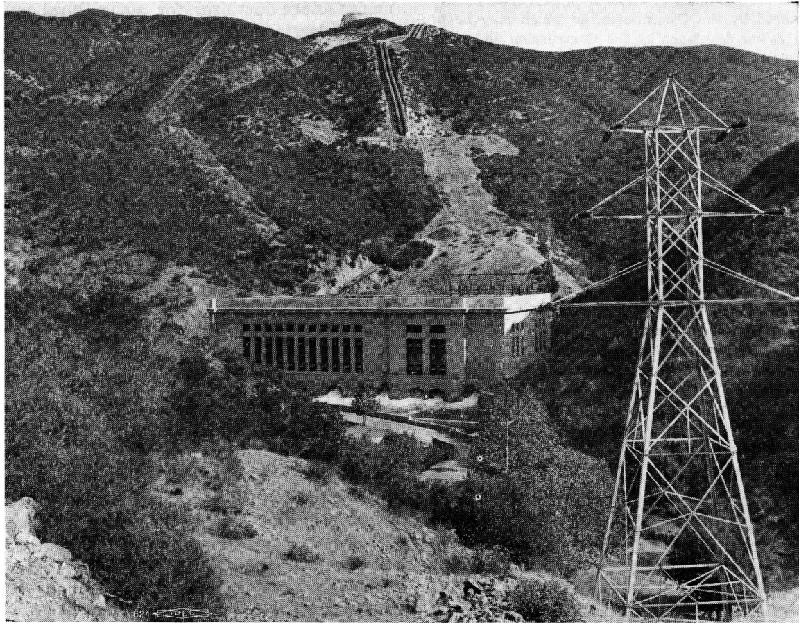
HYDRO-ELECTRIC PLANT NO. 1—LOS ANGELES
