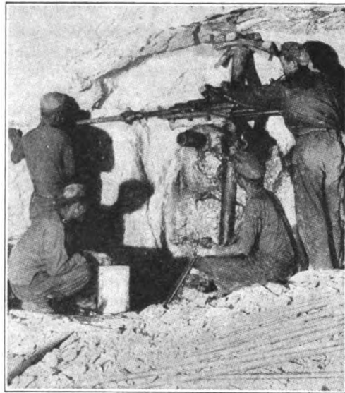
NATIVES RUNNING MACHINE DRILL.
