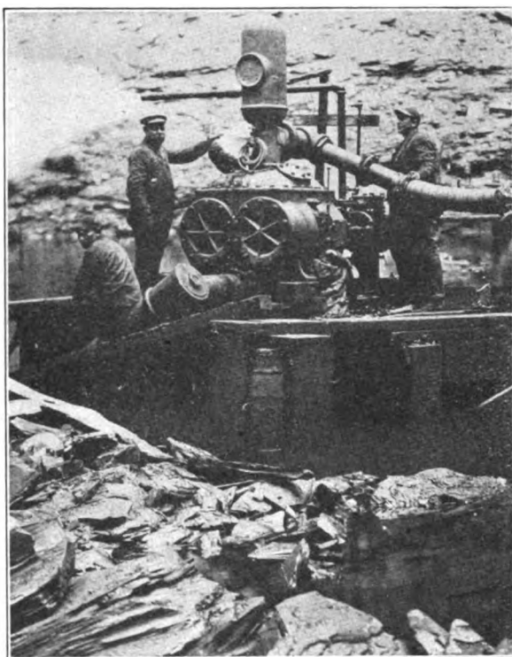
THE PUMPMEN IN THE PIT.
