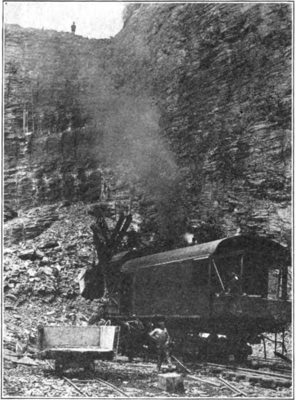
The New Way of Loading Cement Rock with a Sixty-Five Ton Bucyrus Shovel.
