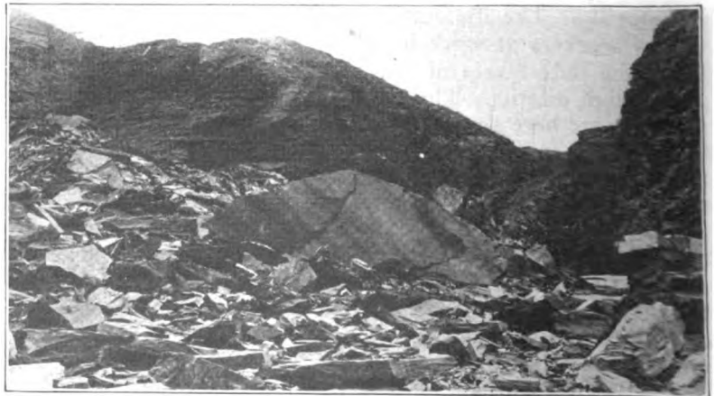
AFTER THE BLAST—2½ TONS OF DYNAMITE—5,000 TONS OF ROCK.
