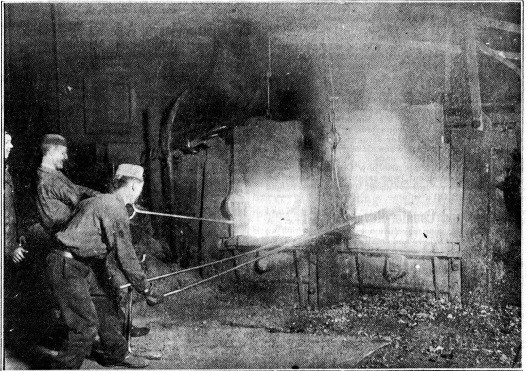
Pulling Out a Lump of White-hot Steel
