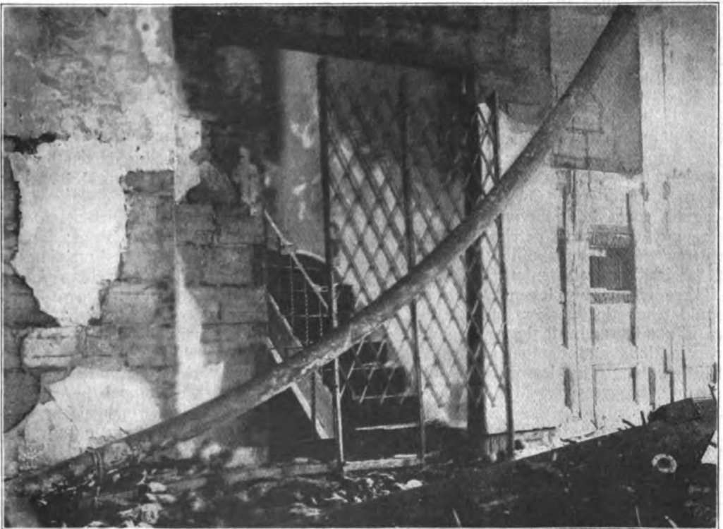
LOCKED GATE THAT PREVENTED ESCAPE.
