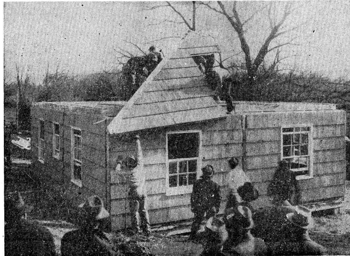
Construction of a pre-fabricated house by members of the CIO United Construction Workers. Gable and roof sections, assembled at factory, can be put together in 3½ hours. Sidney Hillman has used his office in the OPM to refuse to award a contract to the Currier Lumber company, Detroit—which is under contract to the CIO—because of objections from the AFL craft union bureaucrats. Just as Dictator Tobin used to defend the horse against the motor truck, so the AFL fights the use of modern techniques in home construction.
