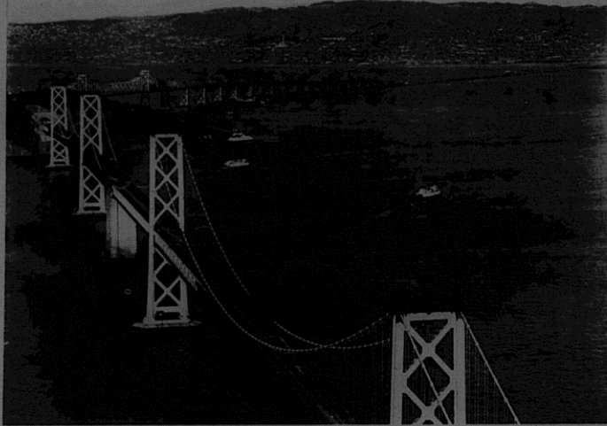
The great San Francisco-Oakland Bay bridge
