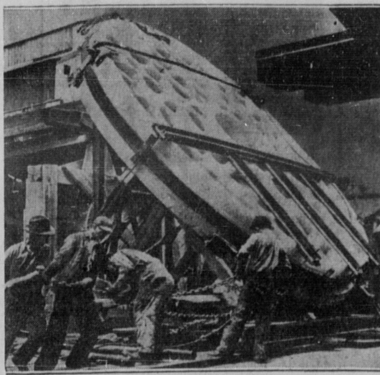
Using house-moving technique, workmen ease the original 200-inch glass disc at Corning, N. Y., through a gap which was cut in a railroad trestle to make way for the twenty-ton telescope eye, biggest in the world. The disc was rendered unfit for service when defects appeared during pouring of the glass, and a second one was made for use at Mt. Palomar, Calif. The original will be put on permanent public display at Corning.
