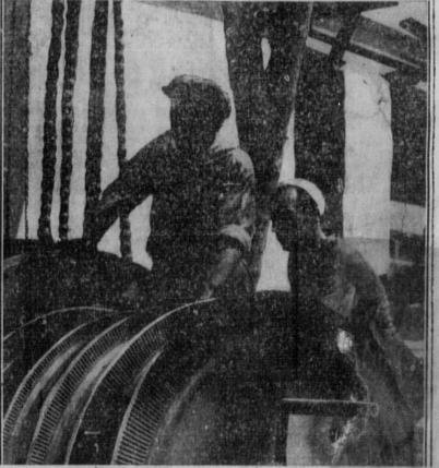
Soviet workers erecting a turbine at Chirchikstrol, off in central Asia near Tashkent near the capital of Uzbekistan. Bringing electricity to the land of the camel, the project will produce more power tlan the famous hydroelectric station on the Dnieper.
