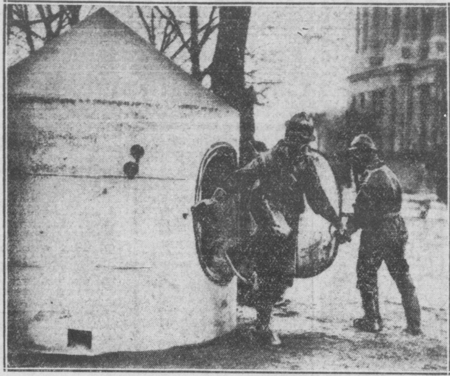
The imperialist French government, competing with America, Japan, Italy and Great Britain, is making extensive preparations for war. Here is a portable metal shelter from gas attacks which was shown recently in Paris by the French Defense Ministry.
