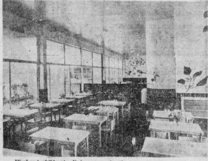
Workers' children's dining room in the new modern school erected by the Communist municipality of Villejuif, near Paris.
