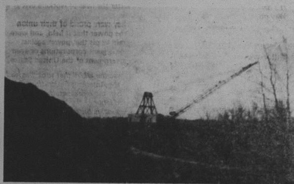
This superstructure houses the "cage," the elevator that lowers men and materials into deep pit mines
