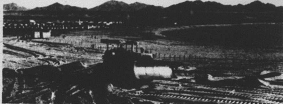
BULLDOZING SITE FOR NEW HOTEL AT SHARM EL SHEIKH
