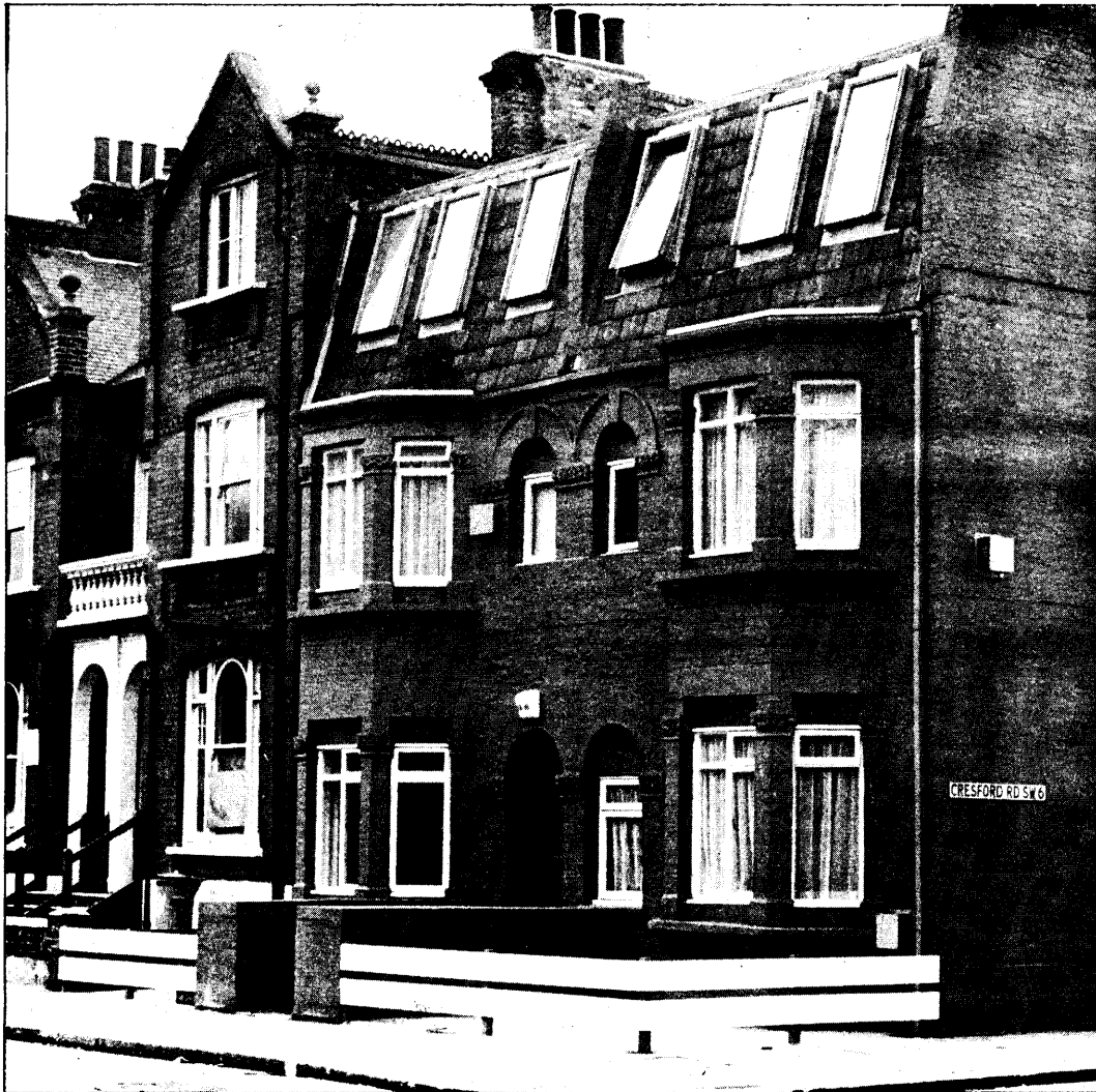
Before and after the grants under the 1969 Housing Act—this time in Fulham. On the left how it used to be. On the right the newly-converted, luxury flats for the middle class.
