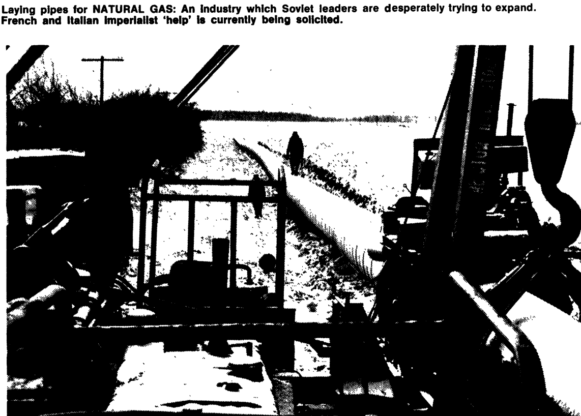
Laying pipes for NATURAL GAS: An industry which Soviet leaders are desperately trying to expand. French and Italian imperialist 'help' is currently being solicited.
