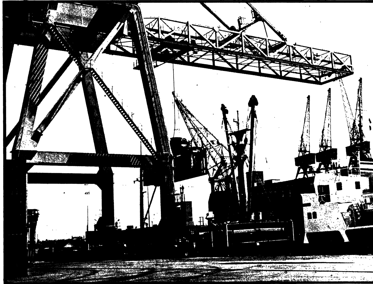
CONTAINER LOADING AT LIVERPOOL: 'Without nationalization,' say dockers, 'developments like this mean the scrap heap for us.'
