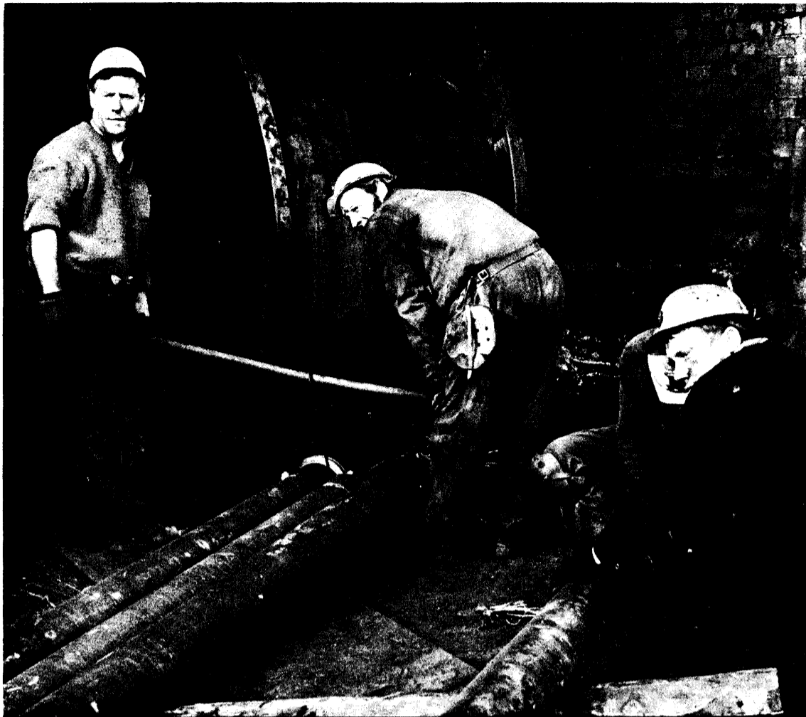
Rescue workers move up pumping gear
