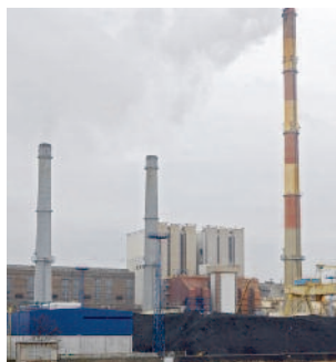
The coal-fuelled Zeran Heating Plant in Warsaw, Poland.
