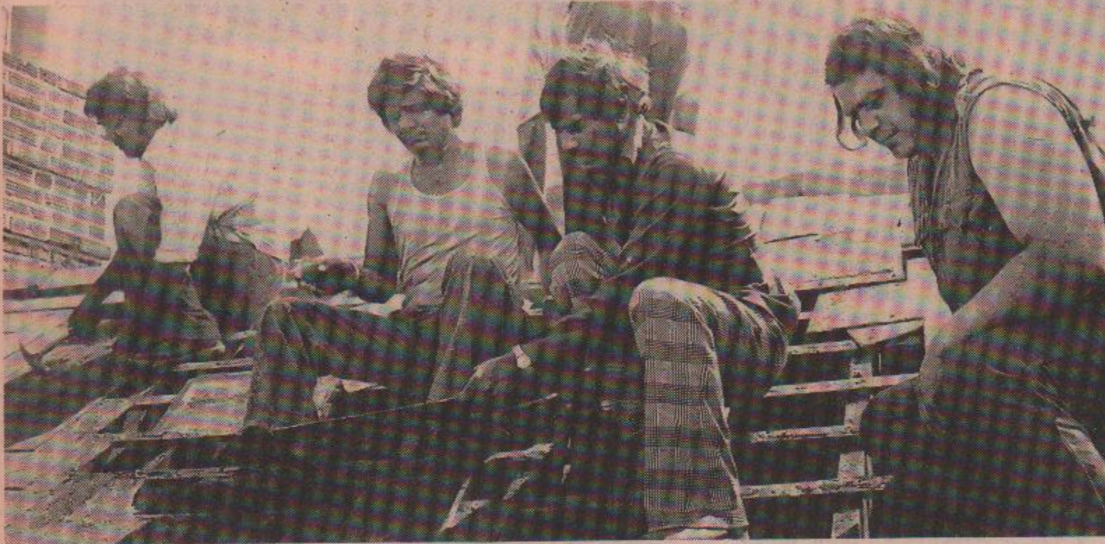
The 'roofers' at work: black and white, united and fighting . . .
