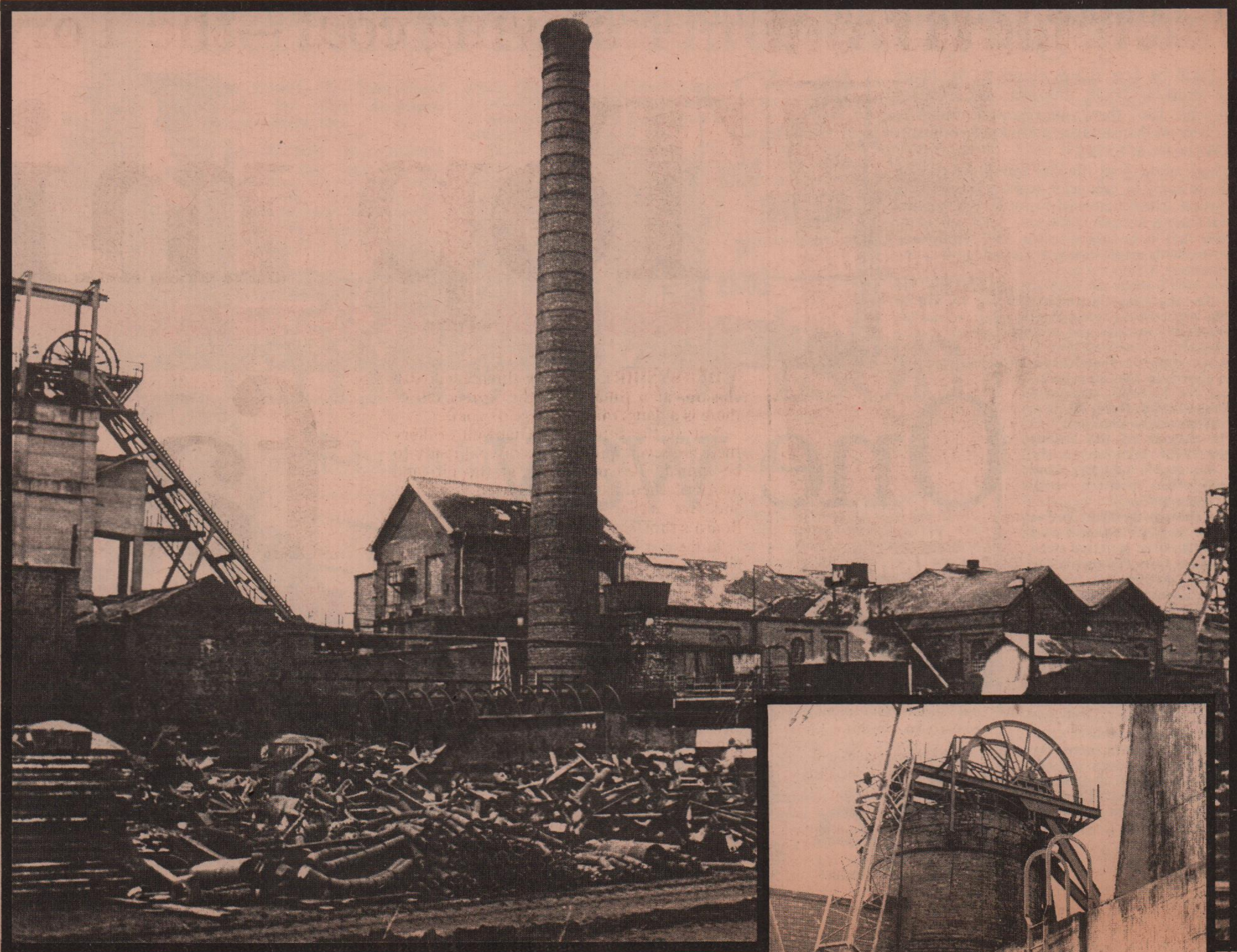
Scrap-iron litters the surface at Glapwell, a pit deliberately run down by the Coal Board. Inset: death's head symbol at Markham, the disaster pit where Glapwell miners will be transferred. Pictures: John Sturrock (Report)
