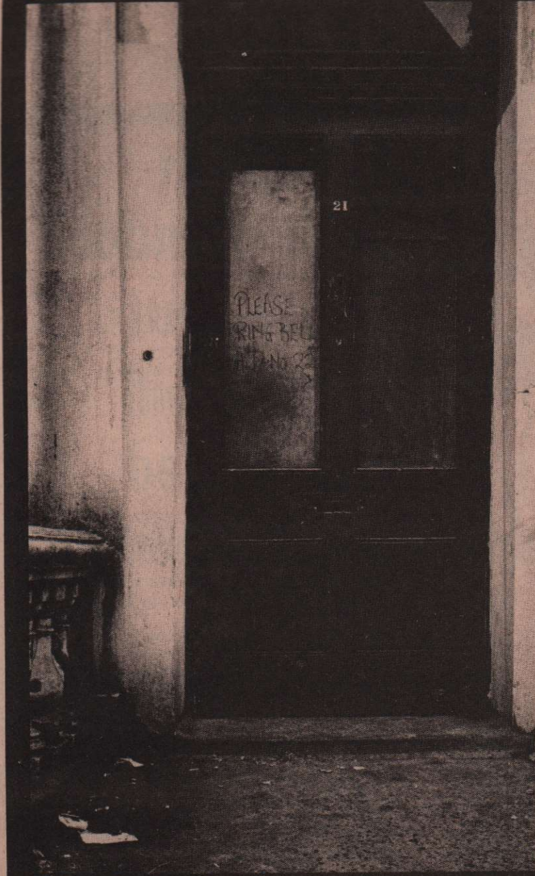
21 Powis Square: waiting for the speculators to start their improvements
