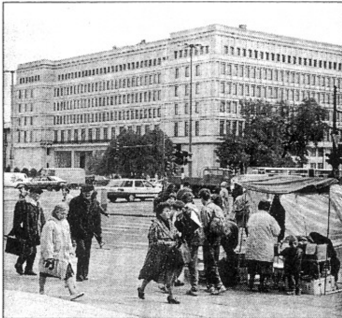
Former Communist Party building that will become the new Warsaw Stock Exchange. New stocks, same bonds.
