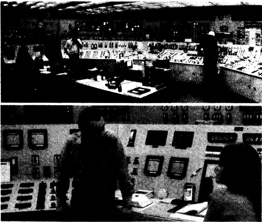
(top) controls at Three Mile Island: above, Fonda and Lemmon
