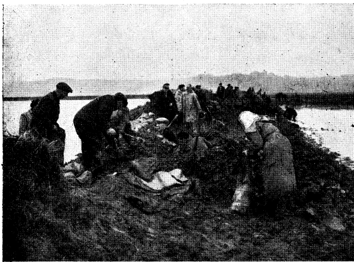
Voluntary workers repairing the breached sea defences on Canvey.
