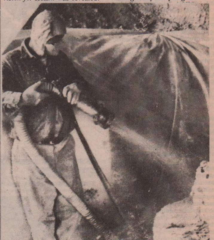
Spraying asbestos
