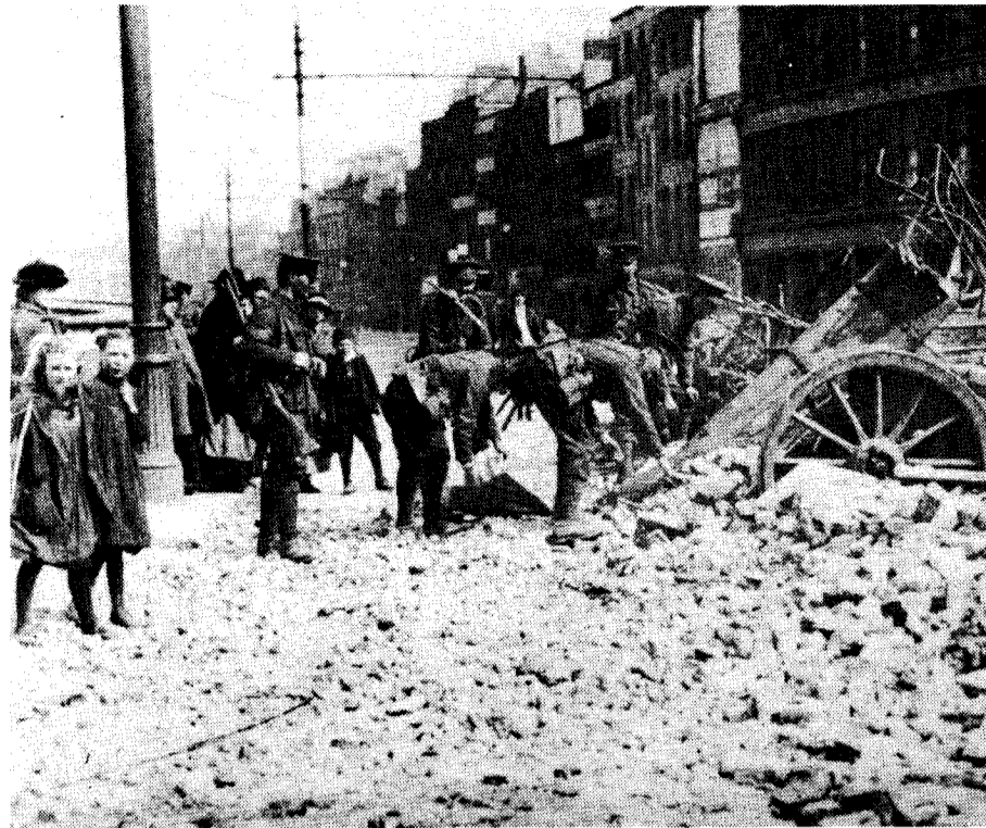
British soldiers among rubble of wrecked buildings in Dublin
