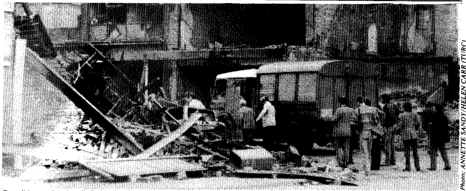
Demolition work in Lozells Road after the fire
