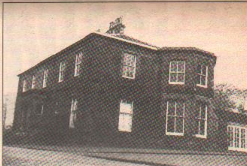
A new private hospital being fitted out at Roundhay in Leeds — just one of the developments the Leeds conference was called to fight.
