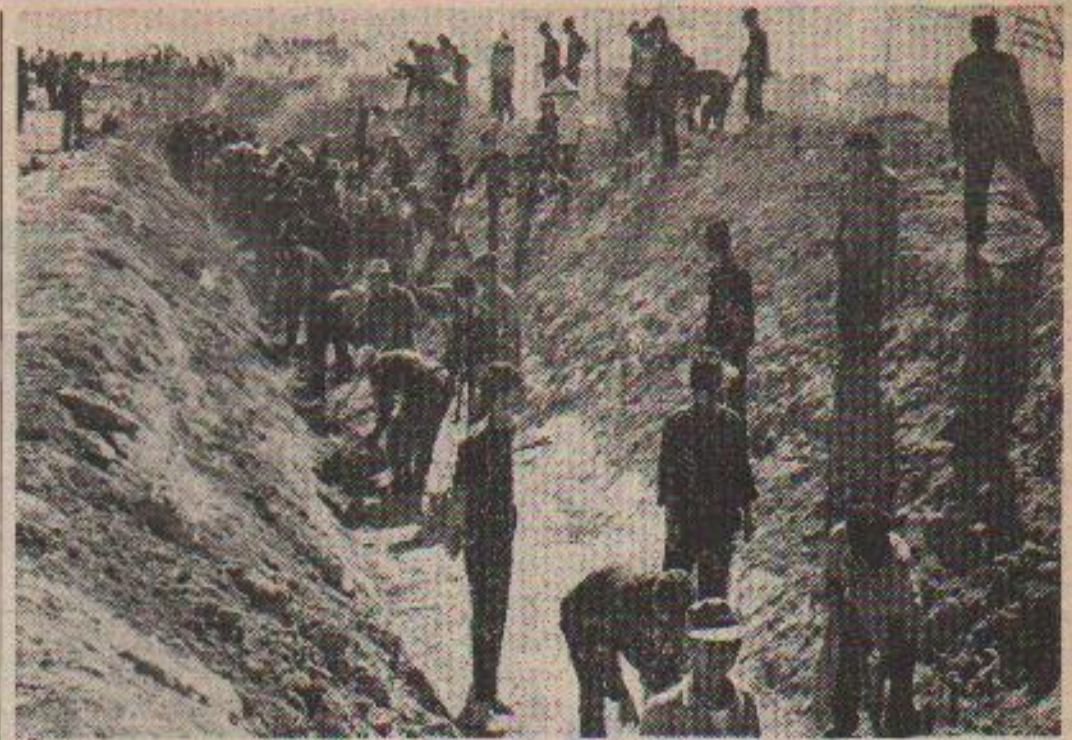
Work in progress on Thieu's pathetic tank-trap trench outside Saigon
