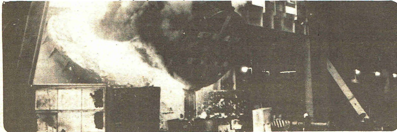
The labour movement must defend all steelworkers' jobs
