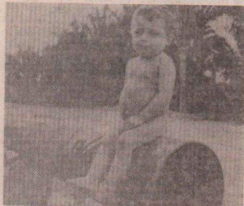
Unfinished pipeline in Mexican jungle
