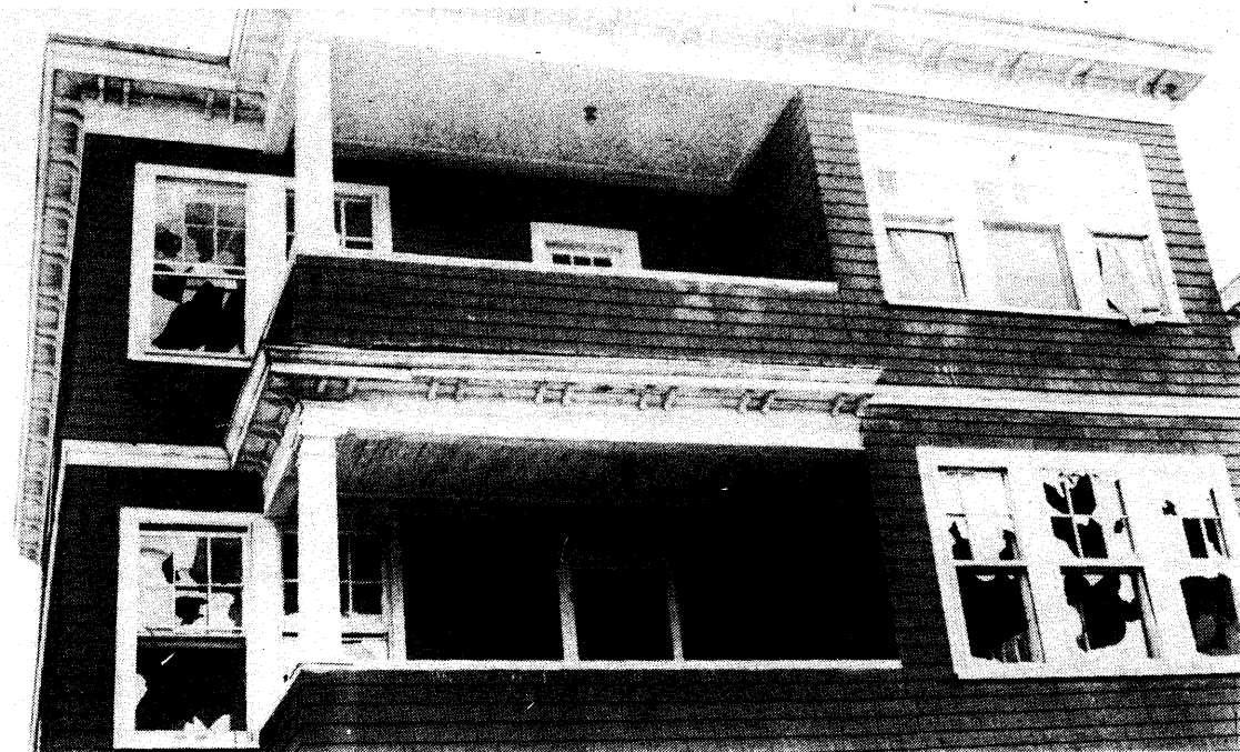
Dorchester housing is abandoned and allowed to deteriorate while landlords push up rents to area residents.
