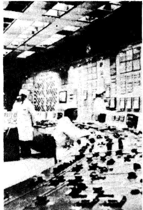
Computerised control room in an atomic power plant near Leningrad.
