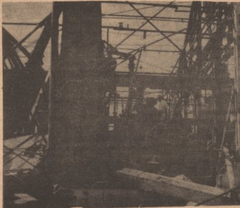
Here is shown 'Ware Chemical' after the explosions.
