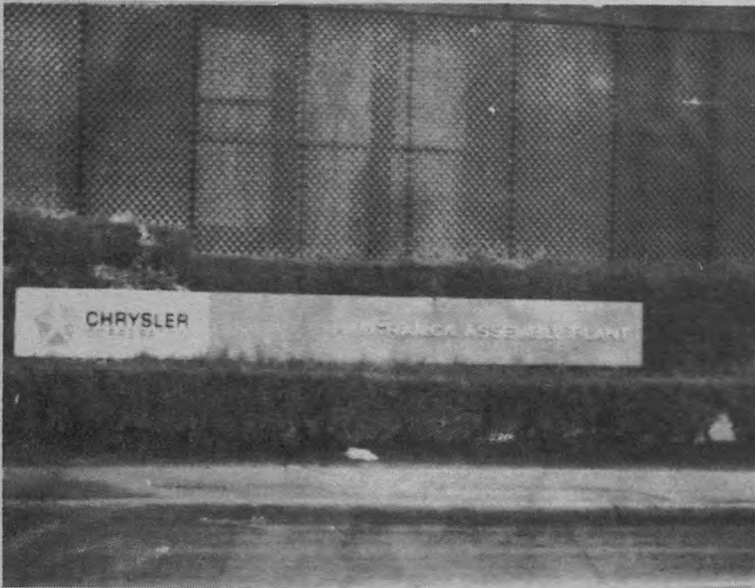
COVERED WINDOWS AT DODGE MAIN
