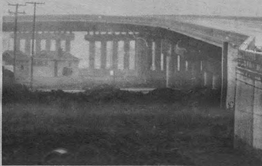
ENTIRE STREET LIFTED INTO THE AIR AT THE LYNCH ROAD ASSEMBLY PLANT, GIVES A MOAT EFFECT.
