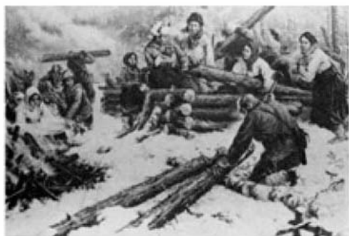
Inhabitants of the guerrilla zone rebuilding houses on sites reduced to ashes by a "punitive" operation
